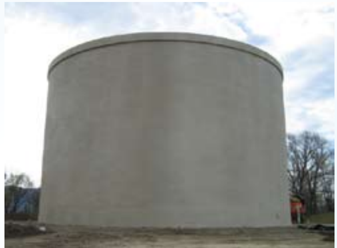
Marne Avenue Tank
