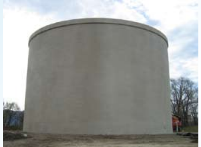
Marne Avenue Tank
